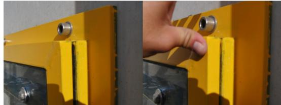
Fig. 7 (left) and Fig. 8 (right): The barrier for the basement window does not close properly
