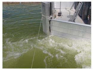
Figure 31: IBS mobile wall system – Demountable flood barriers/dam beams
