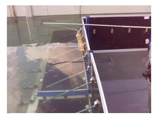
Figure 32: Aquafence – demountable perimeter flood barrier
