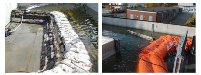
Figure 26: Sandbag system – temporary flood Figure 27: Mobildeich system – temporary perimeter flood barrier consisting of water-filled tubes
