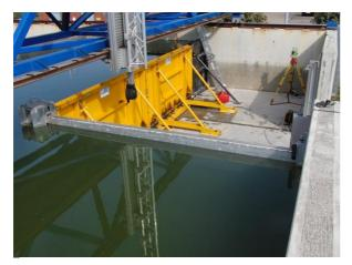
Figure 33: Spring dam system – pre-installed flood barrier
