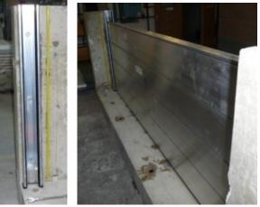
Installation of columns: connection to support with 3 anchor for each column
