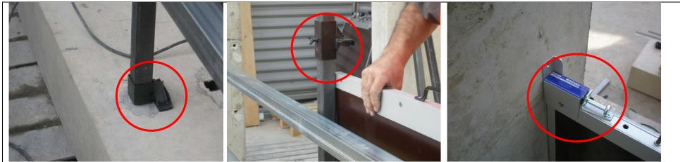
Figure 3 : Flood barrier Collad'eau-Low fastening devices Figure 4 : Flood barrier Collad'eau -Top fastening devices Figure 5 : Flood barrier Collad'eau -Sliding bolts
